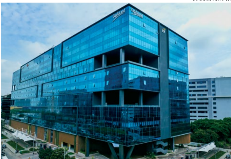
CLINT plans to redevelop International Tech Park Hyderabad (ITPH) in stages over the next seven to 10 years
